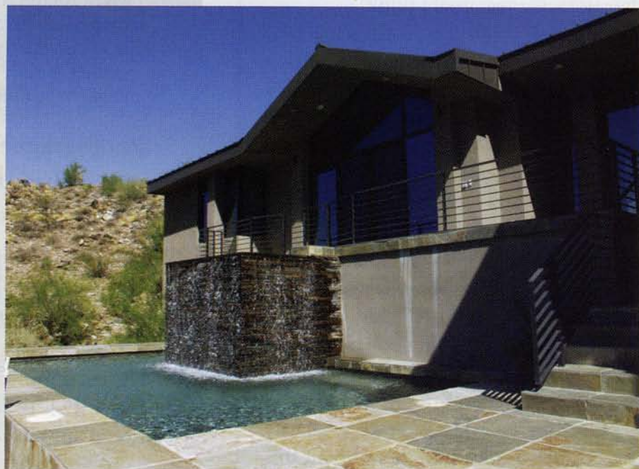
Doubling as a water feature for the swimming pool, the spa is constructed of flat-stacked layers of stone—a more natural look than covering the surface of its walls with broad stone slabs.
